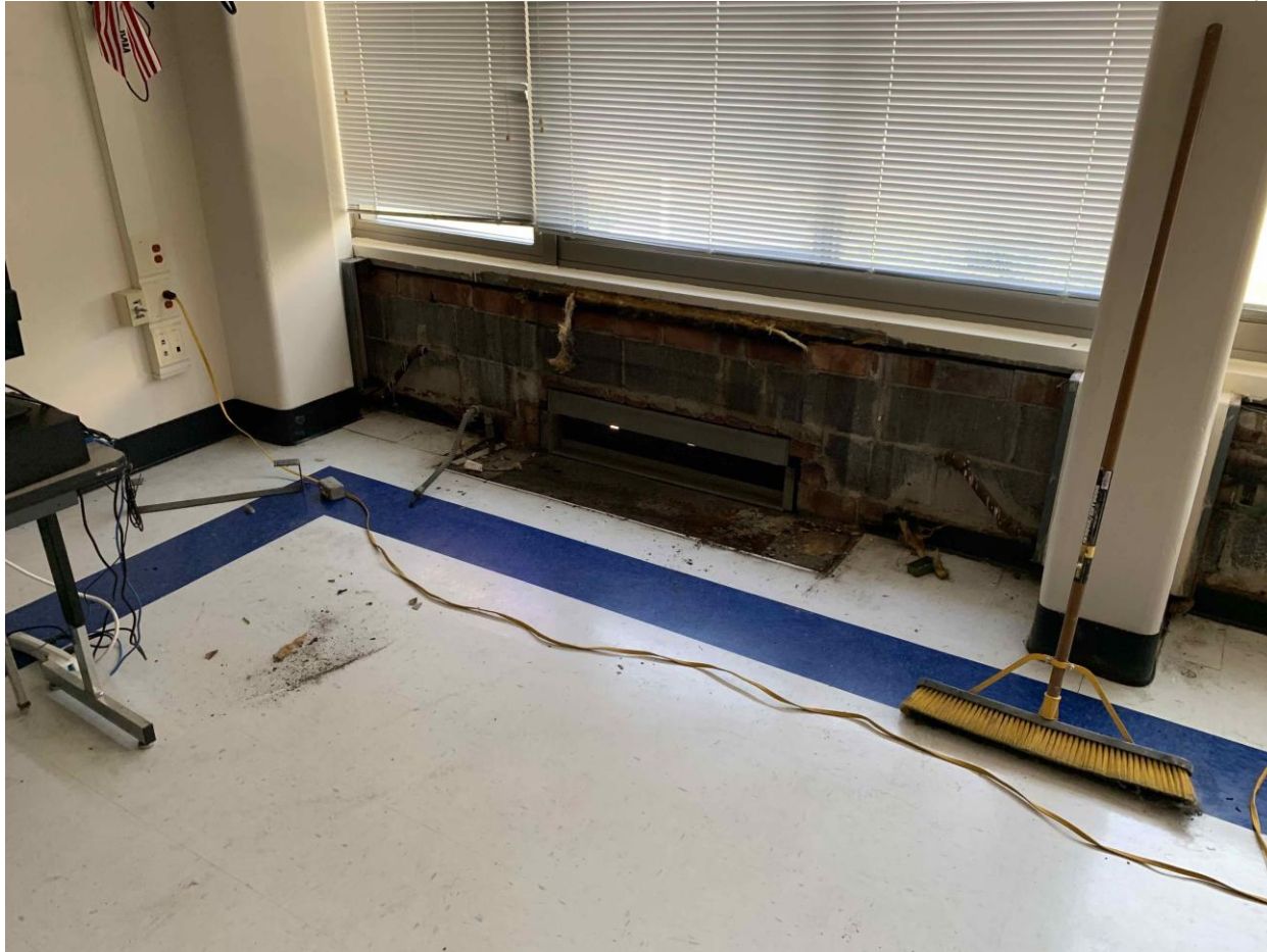
Existing unit ventilators on the third floor have been removed.
