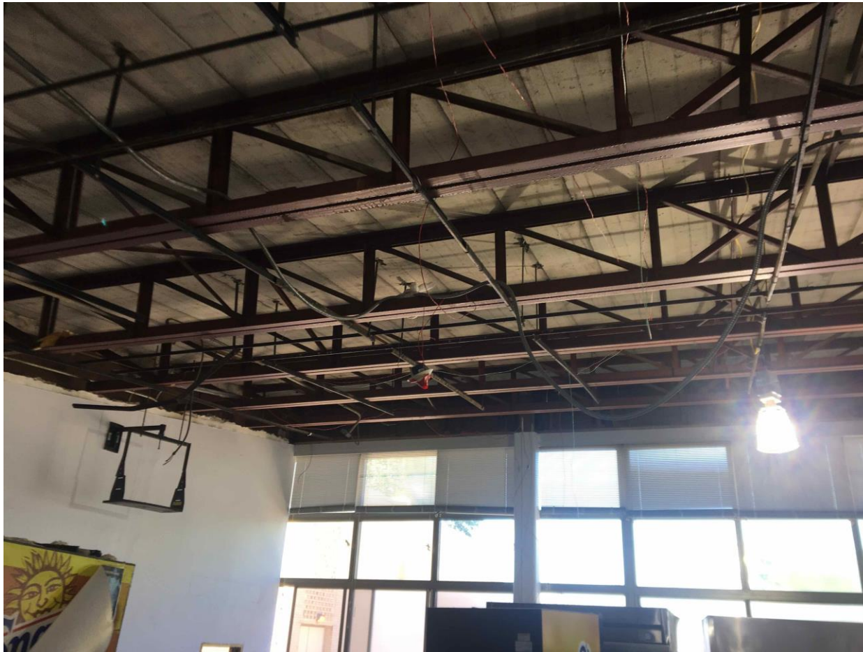
Existing HVAC ducts completely removed in cafeteria A and B.
