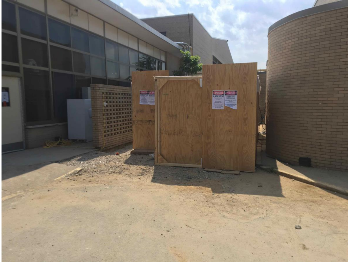
Decontamination chamber set up outside of the cafeteria.
